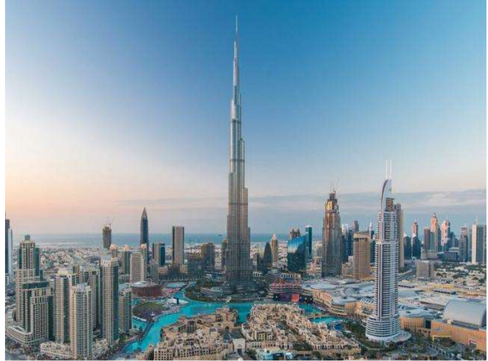
Building a Skyscraper
